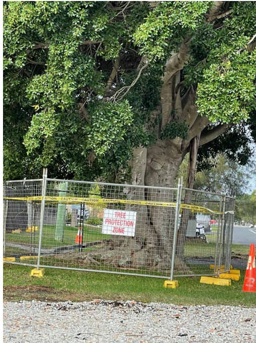
Figure 1. Example of a suitable tree protection fence.
