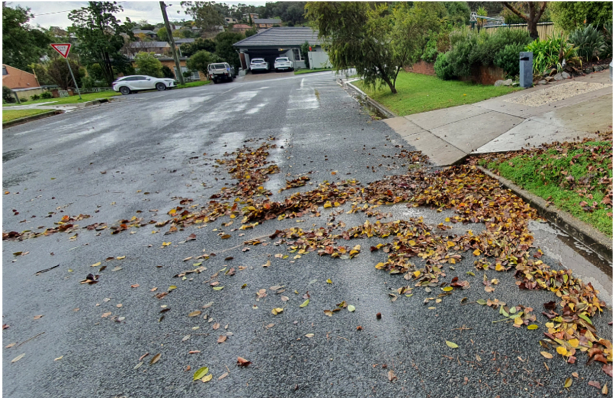
Figure 3. Site visit images from 08-06-2023 showing debris and lengths of flat kerb, causing flows to breach the existing kerb and flow across the one-way cross-fall roads, out of subject site's overland flow catchment.
